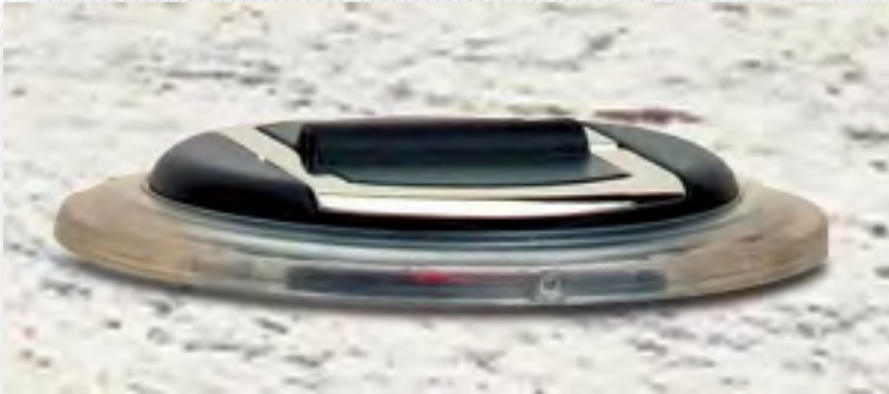
Collapsed Kitchen Outlet Grommet
